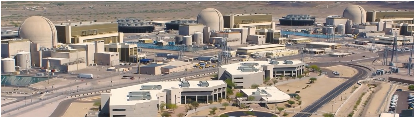
Palo Verde Generation Station
